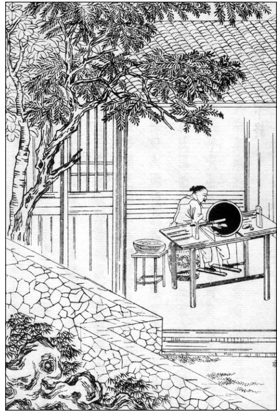
figs. 2 and 3 woodblock prints depicting table-top tu in Tiangong kaiwu 圖二、三 《天工開物》中的砣機式樣
